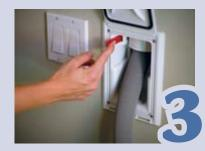
2 ways to turn the vacuum on: **Option 1** - Use the low voltage switch at the inlet.
